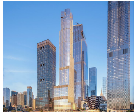
Exterior of 35 Hudson Yards (at the front)
