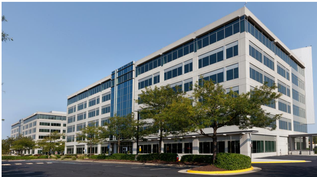
Exterior view of the acquired office building
