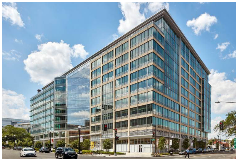
Exterior view of the acquired office building
